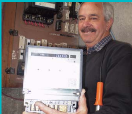
ABOVE: Bay of Plenty Energy contractor Jim Towersey installs a new meter into a business in Whakatane.
