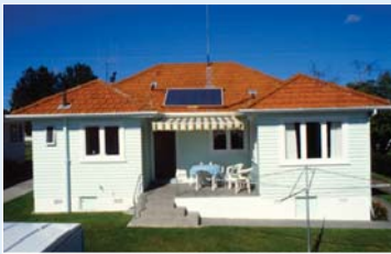
Harnessing solar energy with an efficient solar hot water system installed in your home can reduce your home energy bills.
